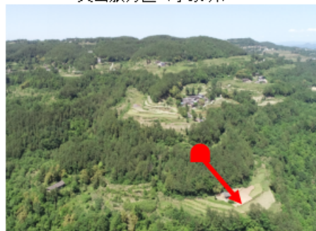
灵山隧道终点
